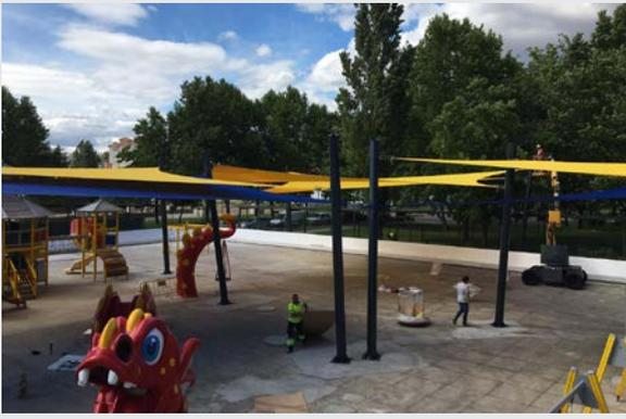
The pillar **Structure** designed to hold the seven Velas consisted of a total of 12 poles S275 dre Ø244 of 6,5 m, with fastenings at different heights depending on the shading design.
